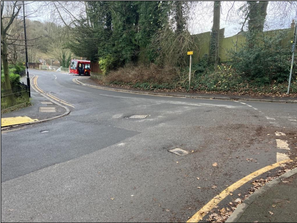
Figure 6: Images of the junction between Hayes Lane and Park Road. The top image is facing Park Road (curving to the right). The bottom image is showing Hayes Lane. The 434 used on the test can be seen turning from Kenley Lane. The driver of this bus cannot see any vehicle that might be approaching from Park Road to the left.
